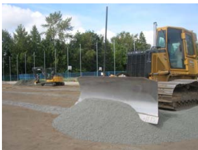
Construction took place over the summer of 2010
