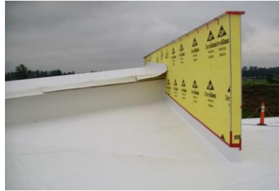
The roof is now 100% complete.
